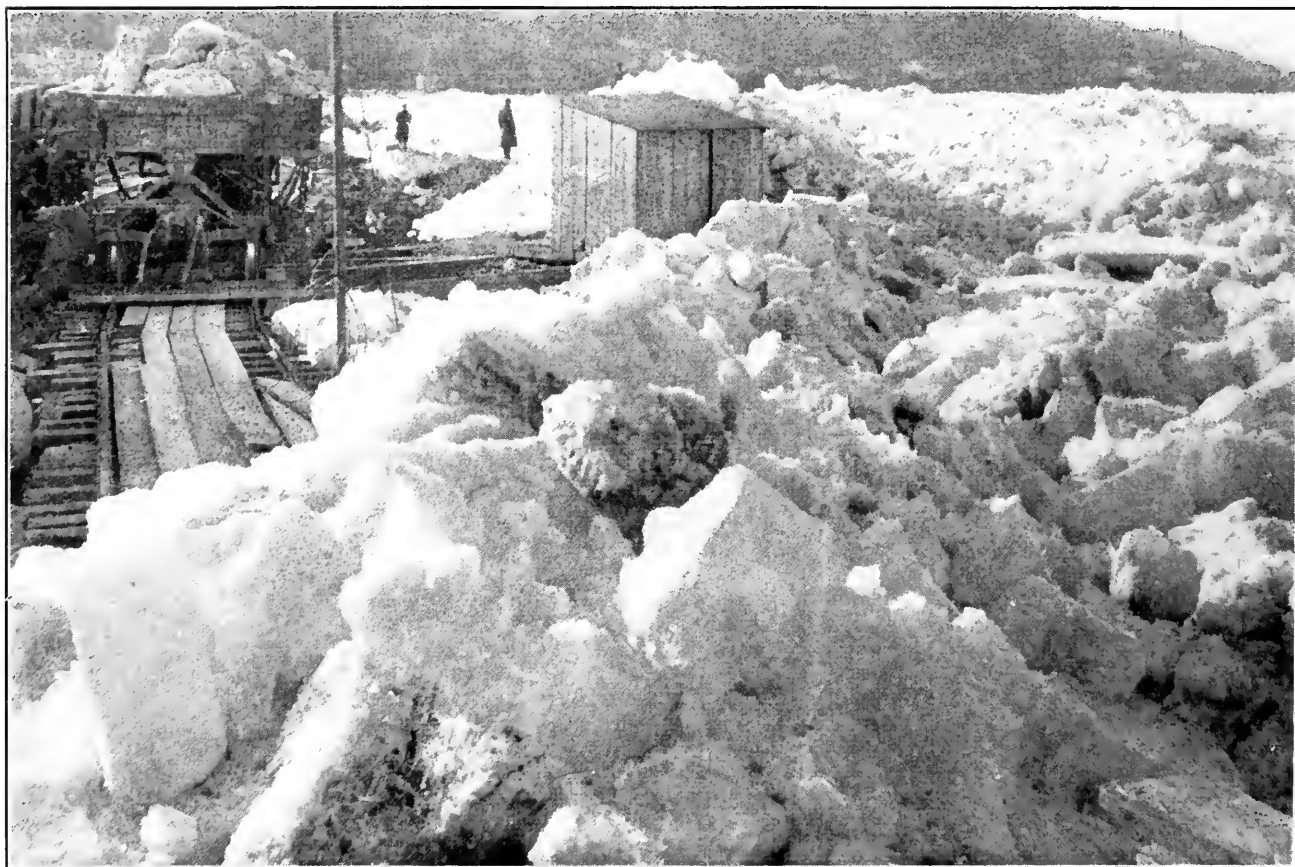
THE COFFER-DAM RESISTING AN ICE JAM LAST MARCH
